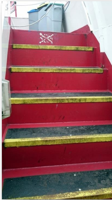
Stairs to Upper Deck
