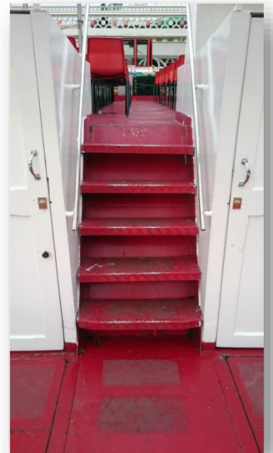
Stairs to Upper Deck
