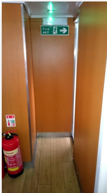
Passage to Gents Urinal and WC
