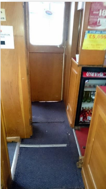
Corridor leading to Saloon Toilet
