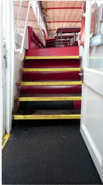
Stairs to Upper Deck
